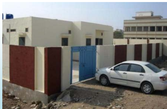
Construction of Basic Health Unit (BHU)
