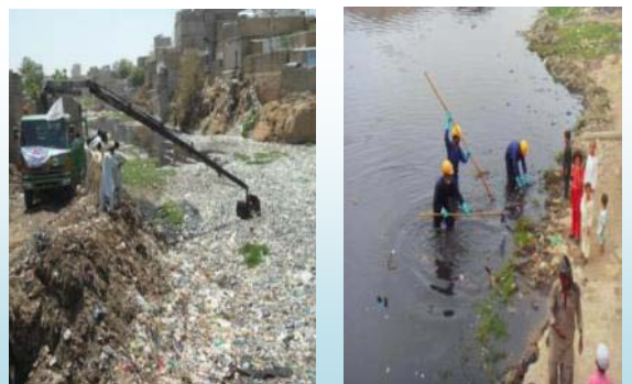
Cleaning of Layari river
