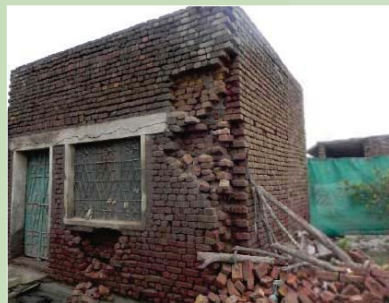
K5 Fired brick with mud mortar Size 1 Room (18X14 ft)
