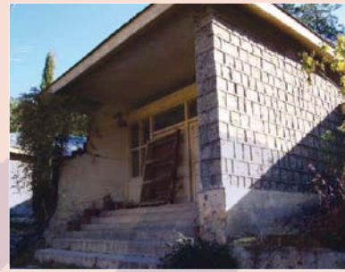
P1 Unreinforced stone masonry C/S mortar Size 1 Room (15X15 ft)
