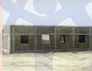
P4 RC Confined brick masonry Size 1 Room (15X15 ft)
