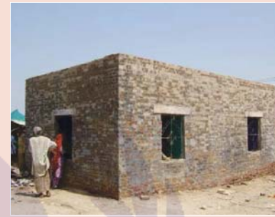
P2 Unreinforced brick masonry C/S mortar Size 1 Room (15X15 ft)
