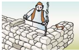
Through stones in stone masonry wall
